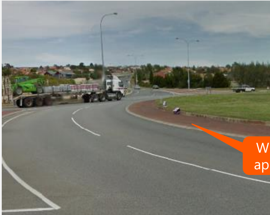
Heavy vehicle wide apron example. Source: MRWA (2015)
