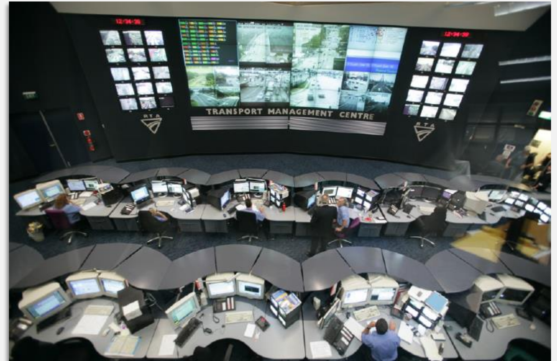
The Traffic Management Centre in Sydney
