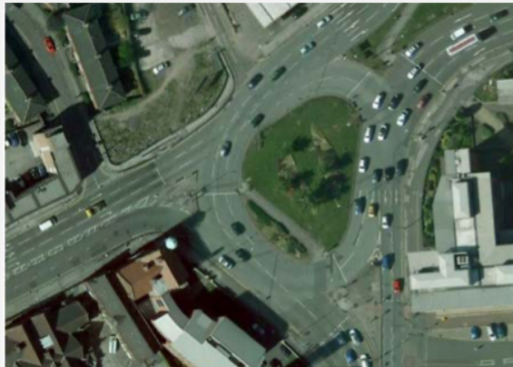
Signalised Roundabout (UK)
