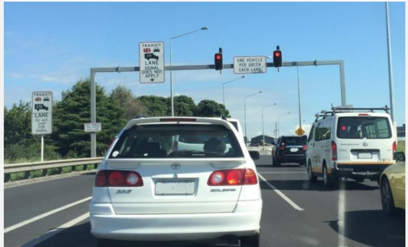
Typical priority lane (left) allowing permitted vehicles to bypass the ramp signals
