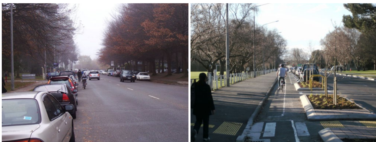
Figure 7.7: Ilam Road before and after bicycle infrastructure was installed
