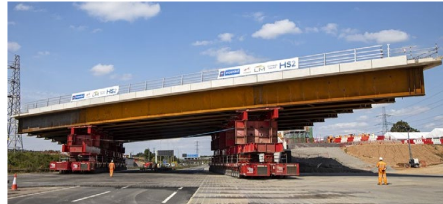
Figure 6.11 – M42 bridge installation
