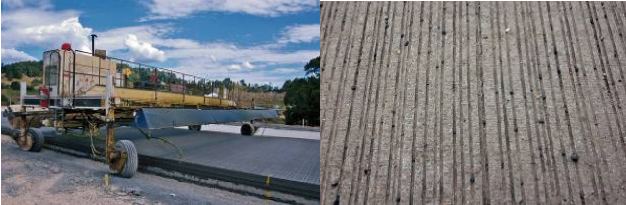
Figure 7.1: Tined concrete surface
