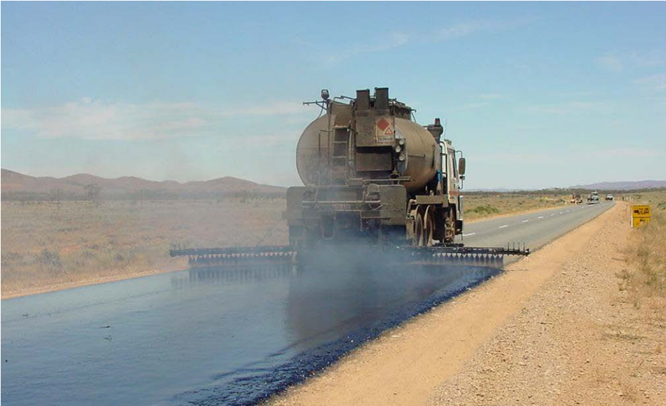
Figure 2.1: Sprayed seal: application of bituminous binder
