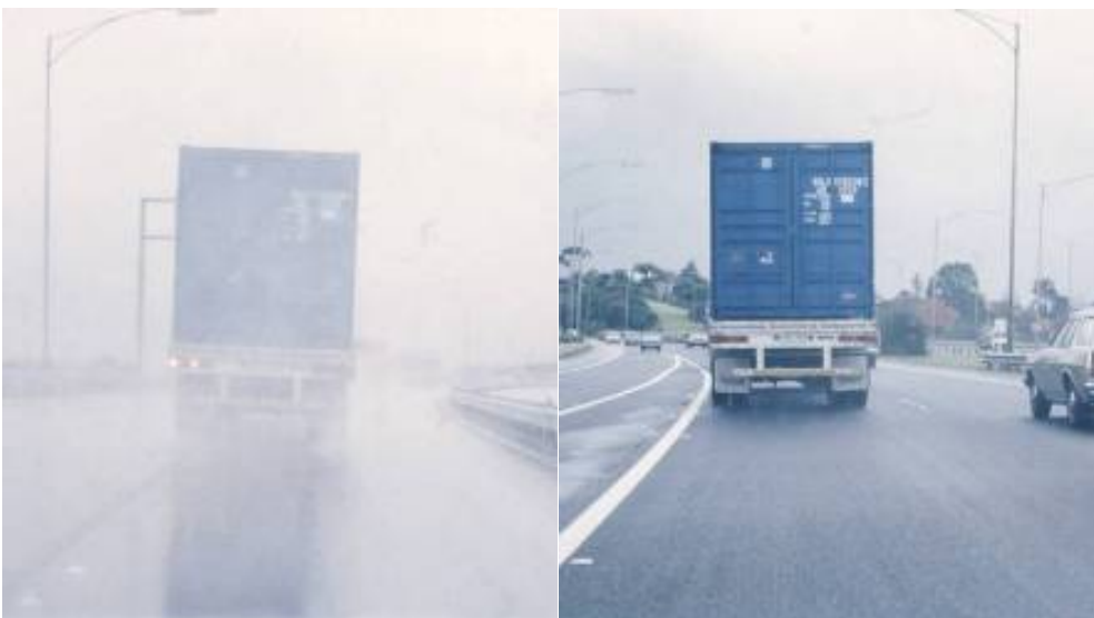
Figure 3.2: Comparative water spray from dense graded asphalt (left) and open graded asphalt (right)
