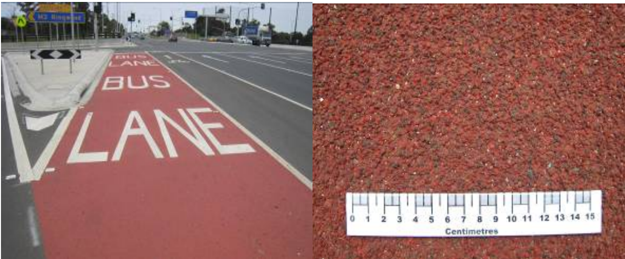
Figure 4.5: Coloured surface treatments using composite slurry (left) and epoxy resin binder with synthetic aggregate (right)
