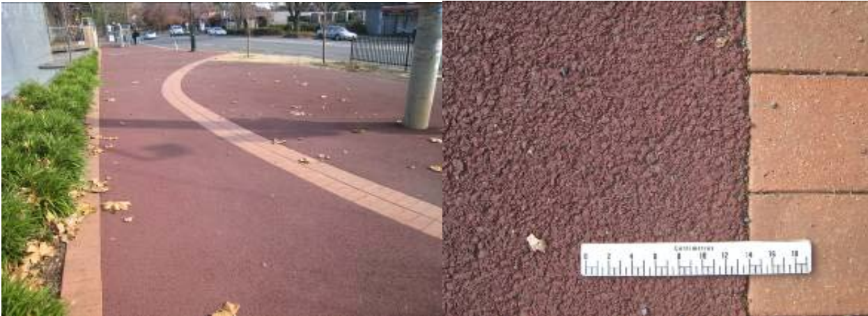
Figure 3.3: Coloured asphalt surface with pigmented binder
