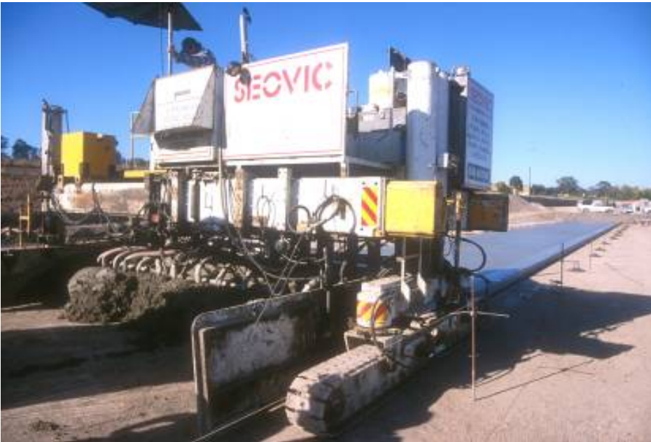
Figure 2.12: Placing plain concrete pavement
