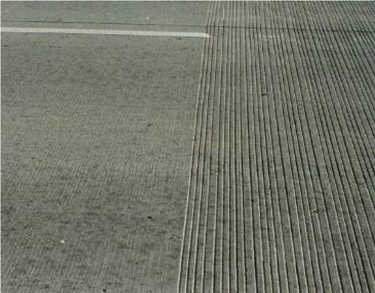
Figure 9.3: Concrete surface texture correction with transverse grooving
