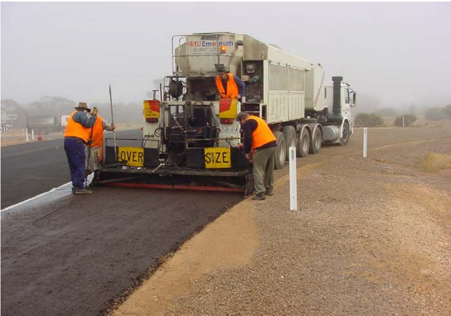
Figure 2.9: Placing bituminous slurry surfacing
