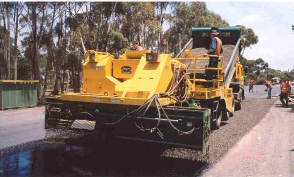
Figure 2.2: Sprayed seal: application of aggregate
