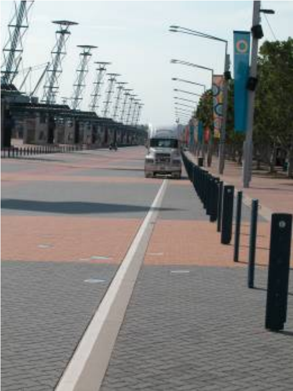
Figure 2.14: Concrete segmental pavement
