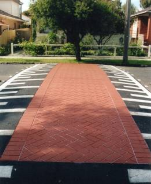
Figure 3.7: Coloured embossed/stencilled asphalt surface
