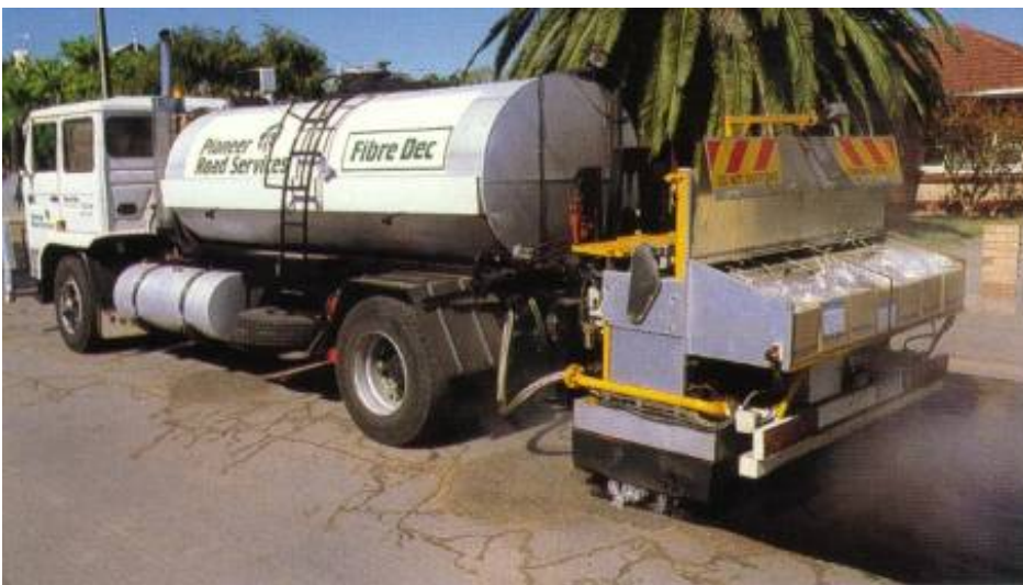
Figure 4.1: Application of fibre reinforced seal
