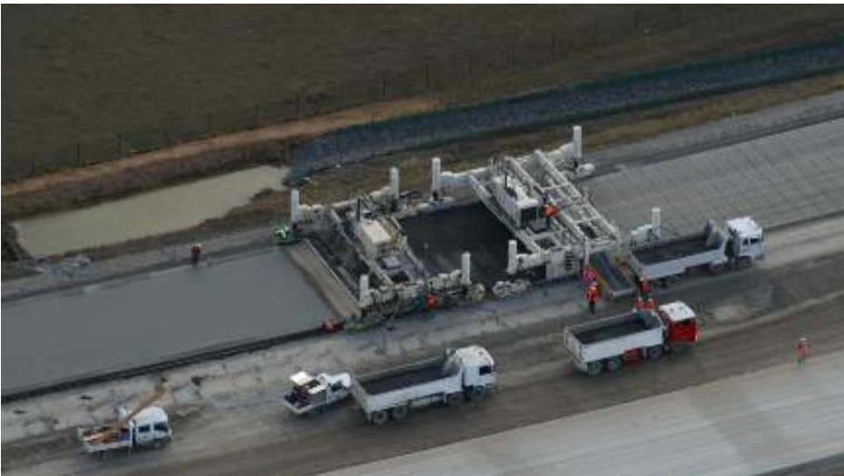
Figure 2.13: Placing continuously reinforced concrete pavement
