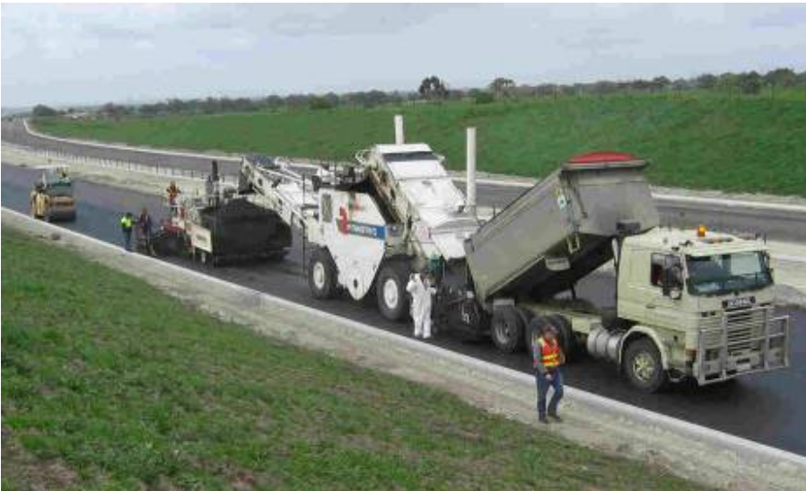
Figure 2.4: Asphalt paving
