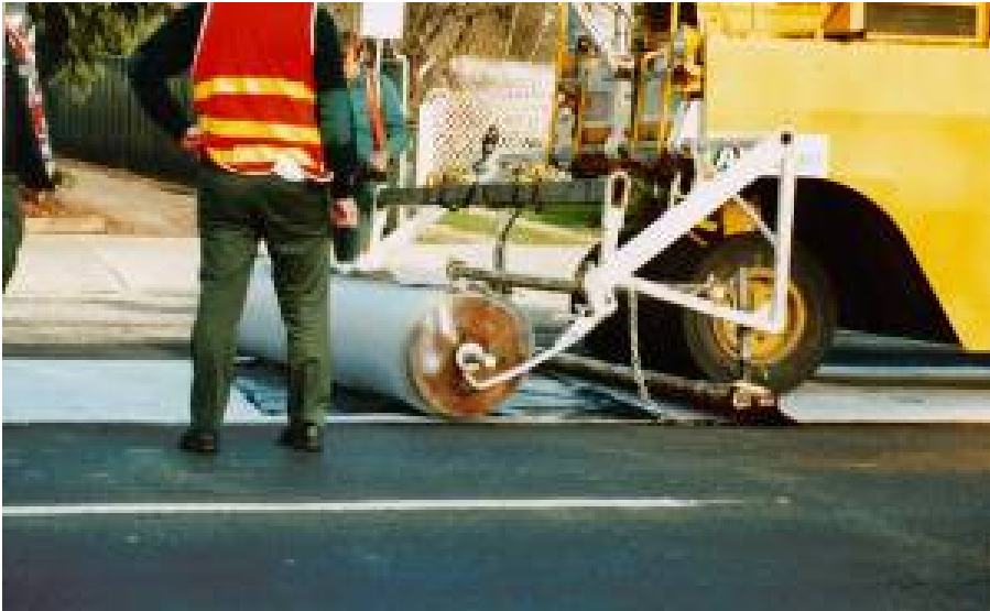
Figure 4.2: Application of geotextile for geotextile reinforced seal
