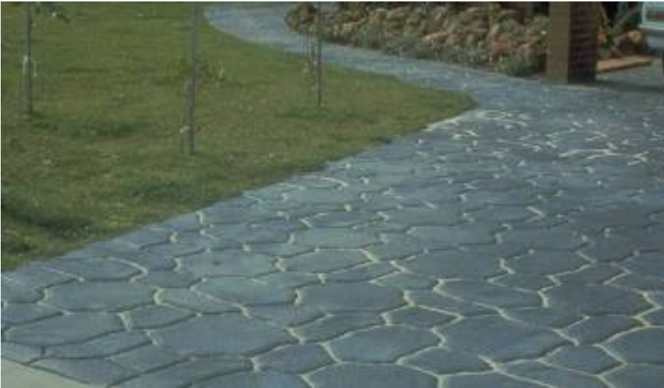
Figure 3.6: Stamped concrete surface
