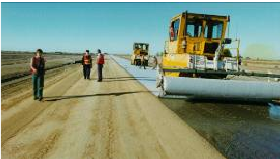
Figure 4.3: Geotextile reinforced seal on a clay pavement
