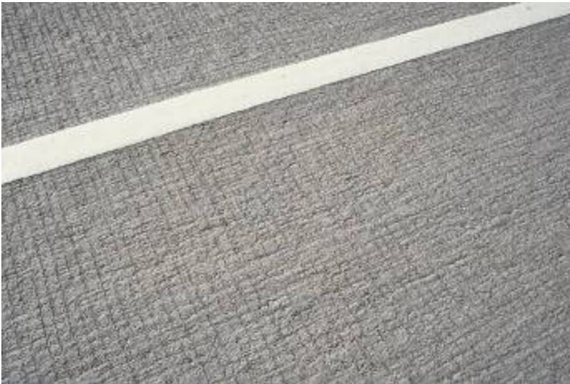
Figure 7.3: Hessian drag followed by transverse tine
