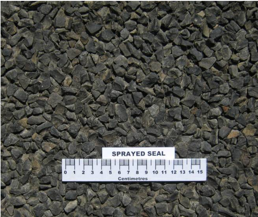
Figure 2.3: 10 mm sprayed seal surfacing
