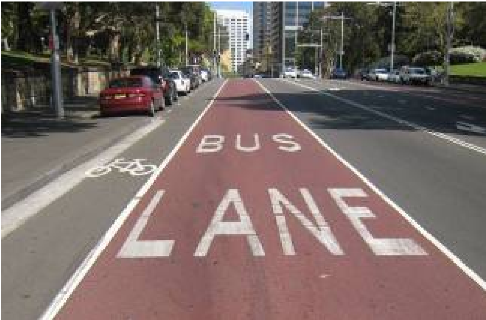
Figure 3.1: Delineation of bus lane with coloured asphalt surface
