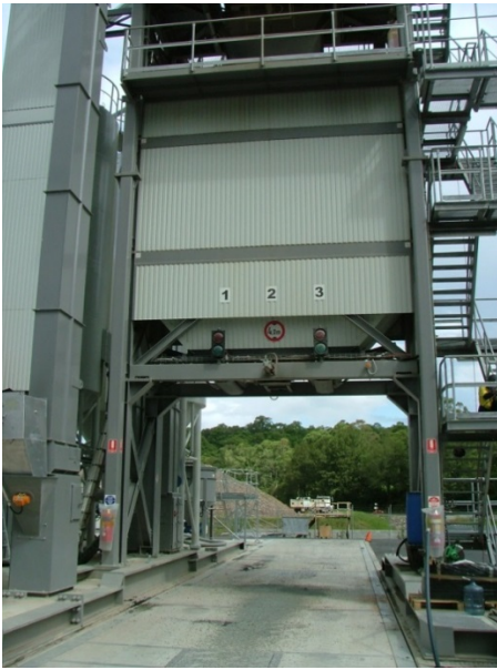
Figure 5.11: Asphalt surge bins
