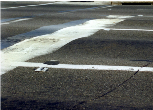
Figure 4.12: Typical rutting
