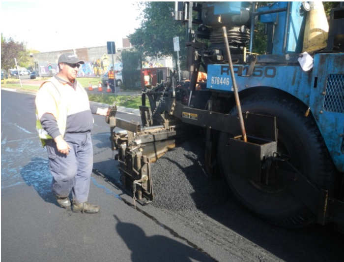
Figure 1.2: Asphalt paver in operation
