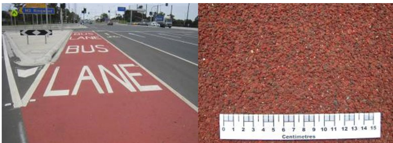
Figure 3.15: Coloured surface treatment incorporating epoxy resin binder and synthetic aggregate
