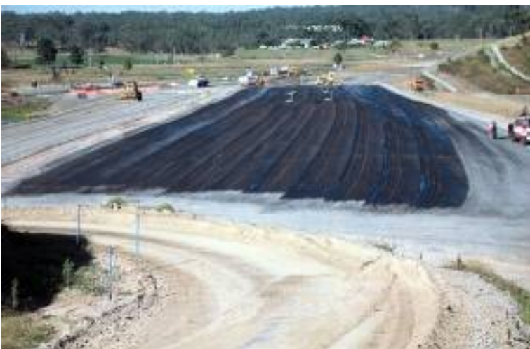
Figure 3.17: Dust laying techniques for other engineering works
