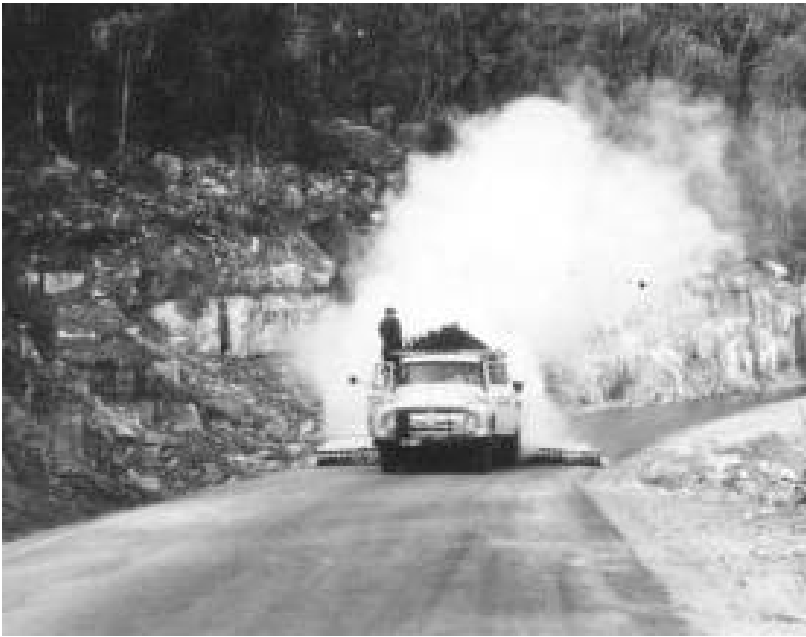
Figure 1.4: Applying sprayed seal binder circa 1960s
