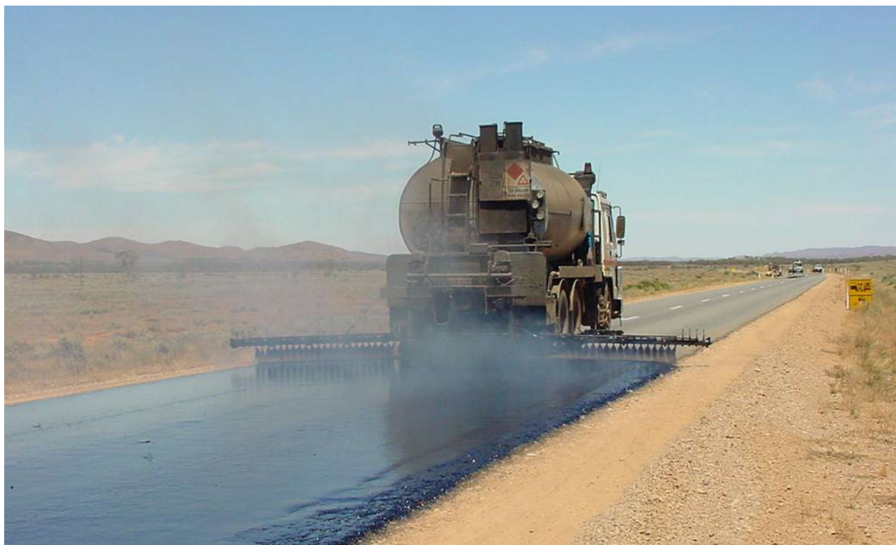
Figure 1.2: Spraying bituminous binder
