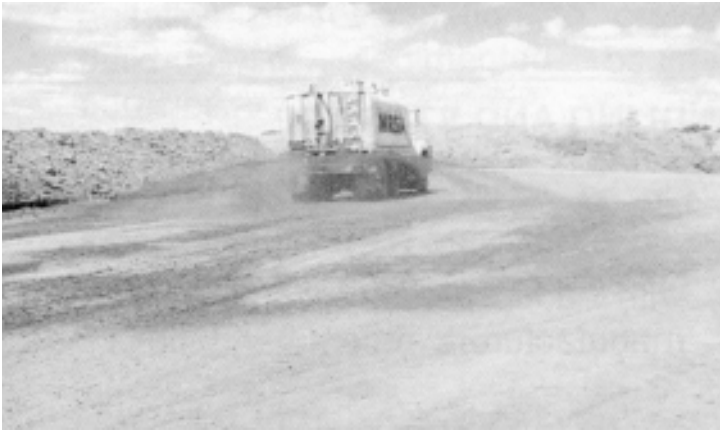
Figure 3.16: Dampening down dusty surface
