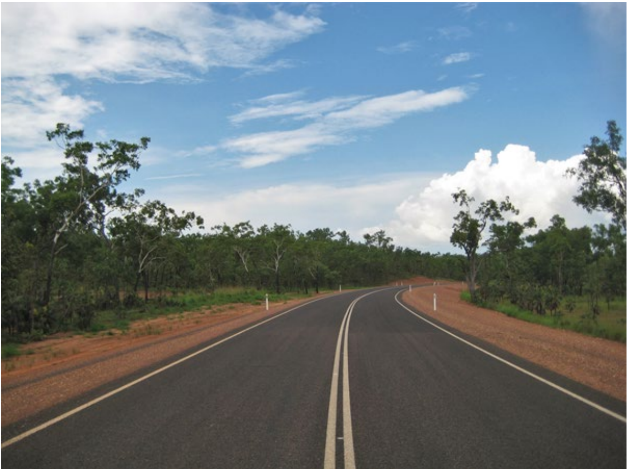
Figure 1.1: Sprayed seals are an important element of the Australasian road system
