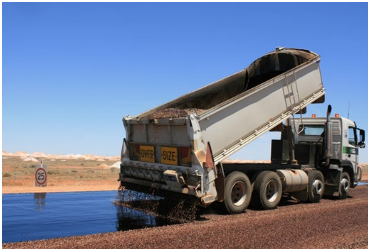
Figure 1.3: Spreading aggregate
