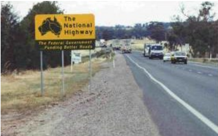
Figure 2.1: High-volume traffic on a sprayed seal pavement
