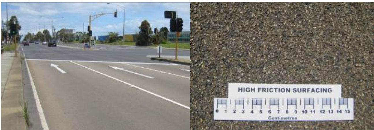
Figure 3.14: High-friction surface treatment
