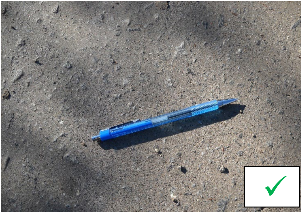
Figure A 1: Examples of well-prepared granular pavements
