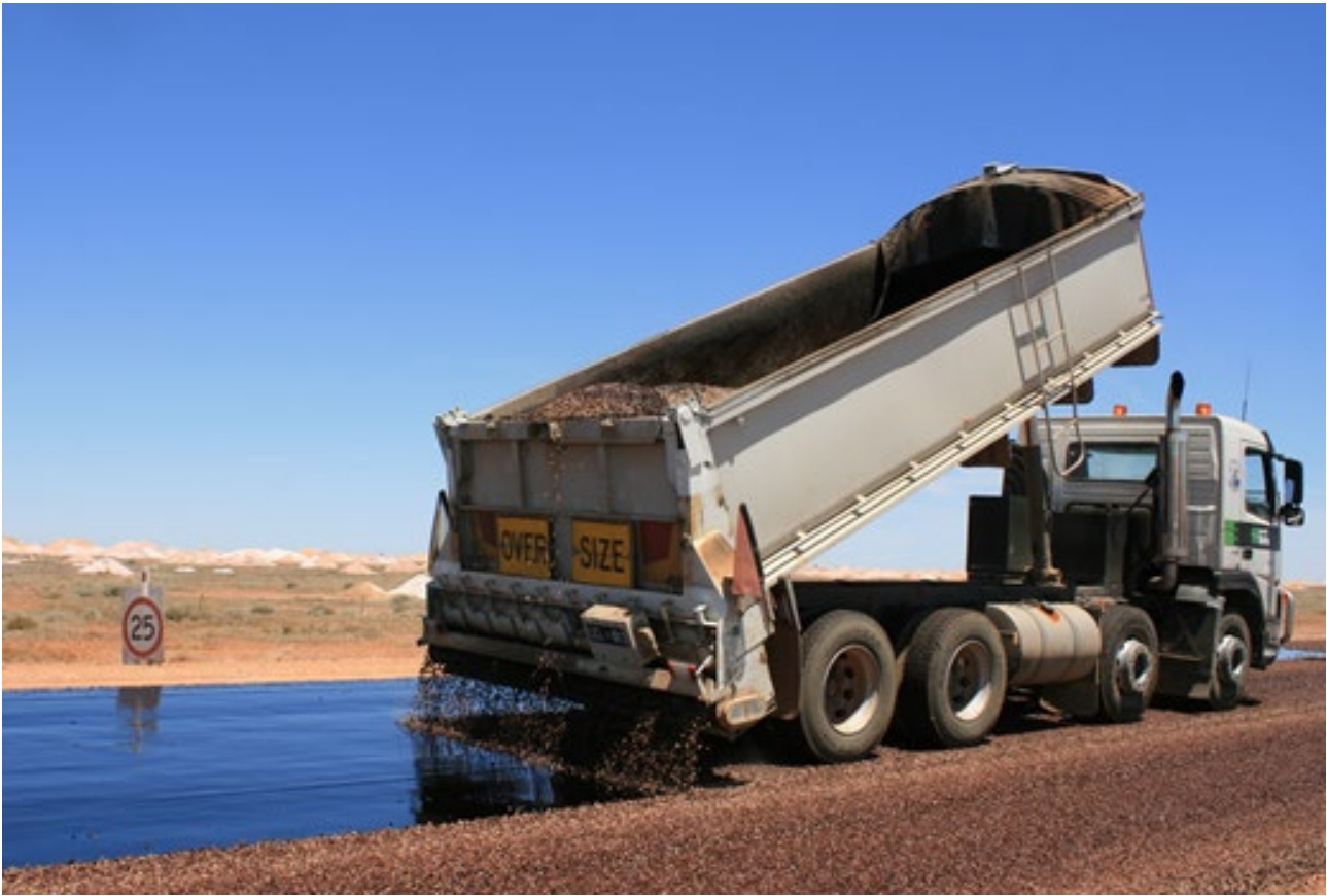
Figure 1.3: Spreading aggregate
