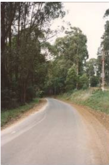
Figure 2.4: Sprayed seal pavement in a damp, cool environment
