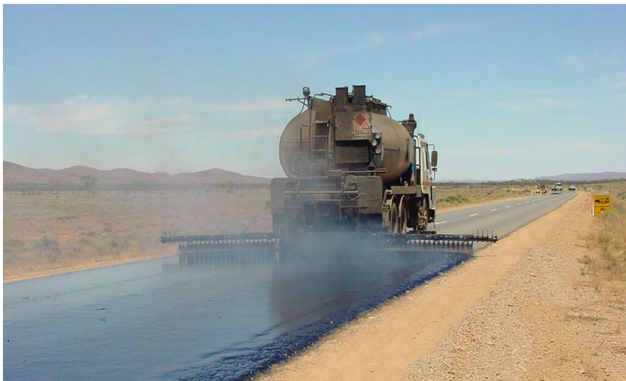
Figure 1.2: Spraying bituminous binder
