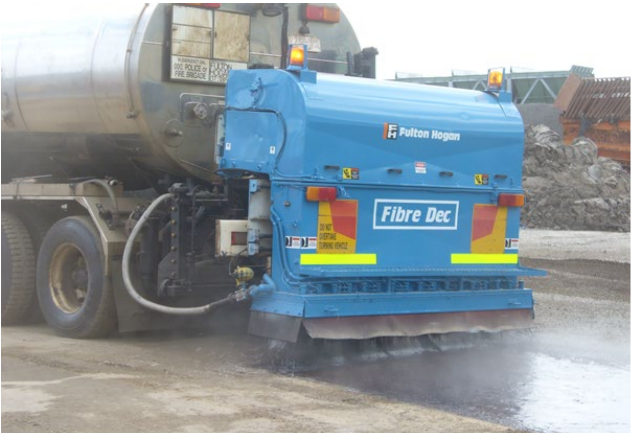
Figure 3.11: Application of binder and fibre for fibre reinforced seal
