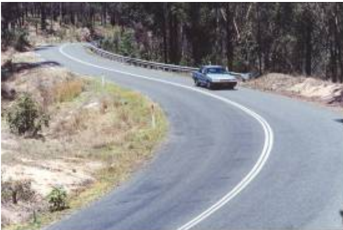
Figure 2.2: Low-volume traffic on a sprayed seal pavement
