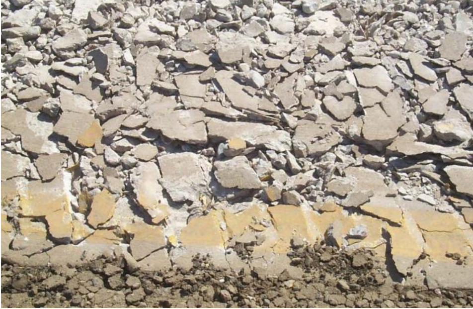
Figure 8.11: Concrete pavement after being rubblised using a multi-headed breaker
