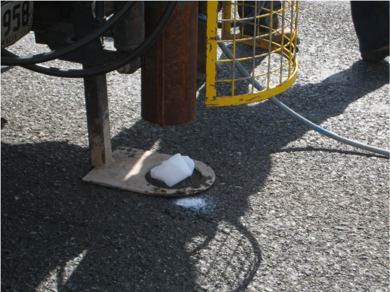
Figure 5.3: Coring of bound materials using compressed air and dry ice
