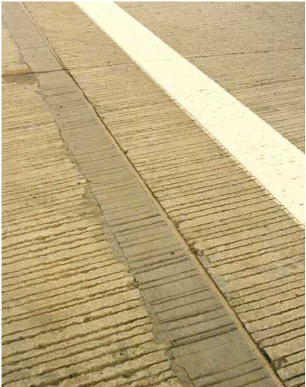
Single-sided spall repair
