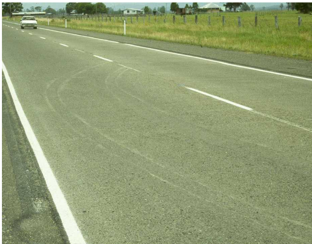
Repaired area after 25 years
