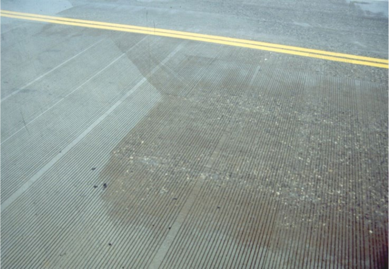
Figure 8.5: The surface of a bridge deck which has been longitudinally ground and transversely grooved
