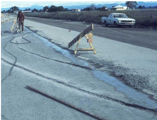
Sawing along each side to provide vertical edges
