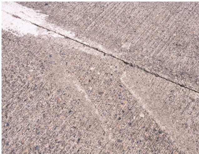
Acute corners must be avoided by squaring all joints and junctions as shown
