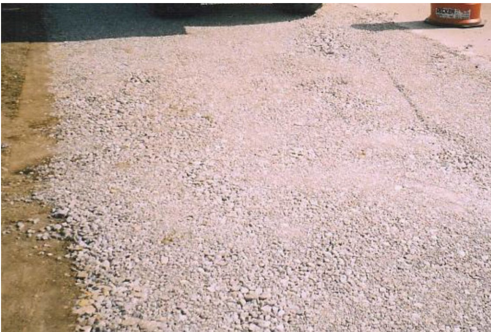
Figure 8.12: Rubblised pavement surface after rolling
