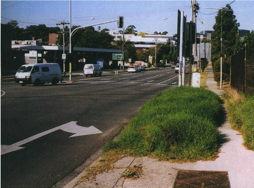
Figure 7.20: The path to pedestrian signals is narrow and overgrown
