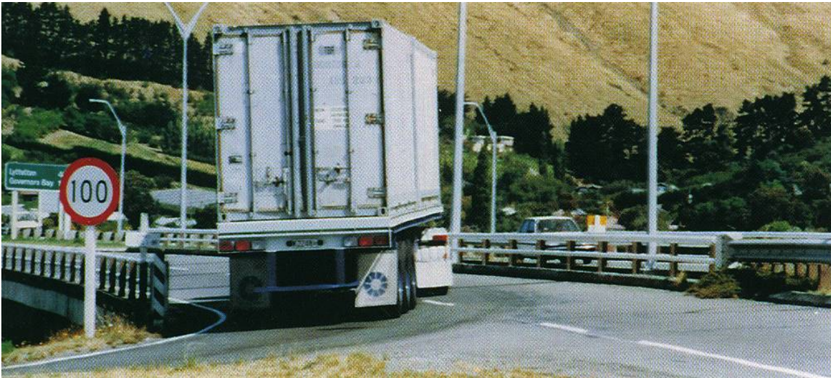
Figure 7.6: Large trucks enter Tunnel Road
