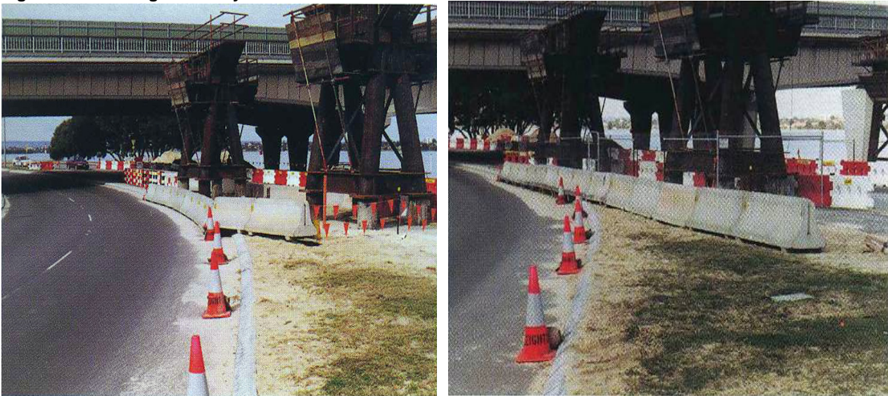
Figure 6.3: Realigned safety barrier
