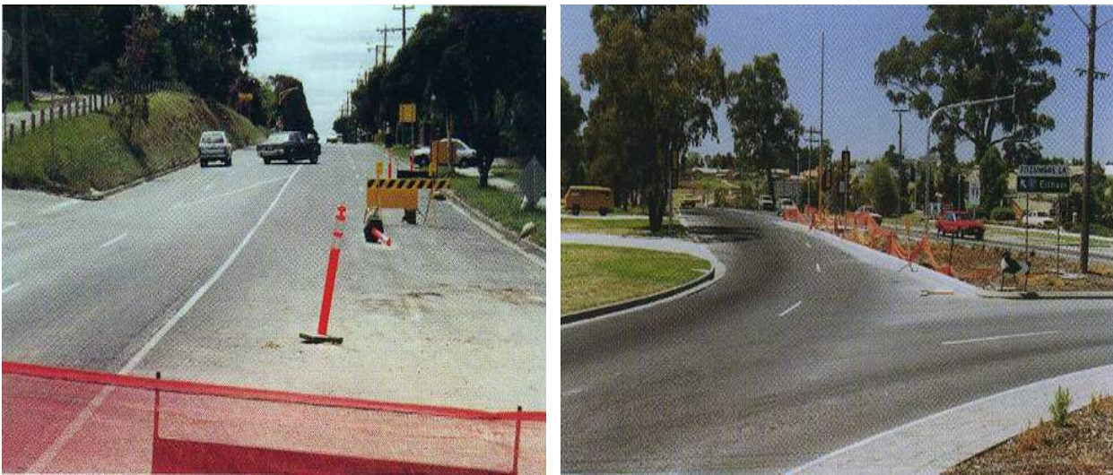
Figure 6.4: Confusing line markings
