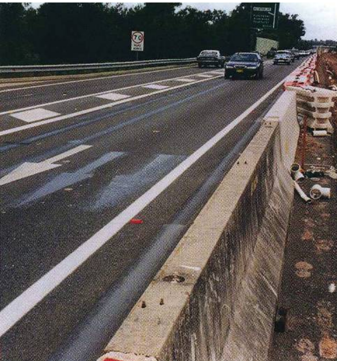
Figure 7.17: Blacked-out pavement lines and arrows are confusing especially at night-time; barriers overlapped incorrectly
