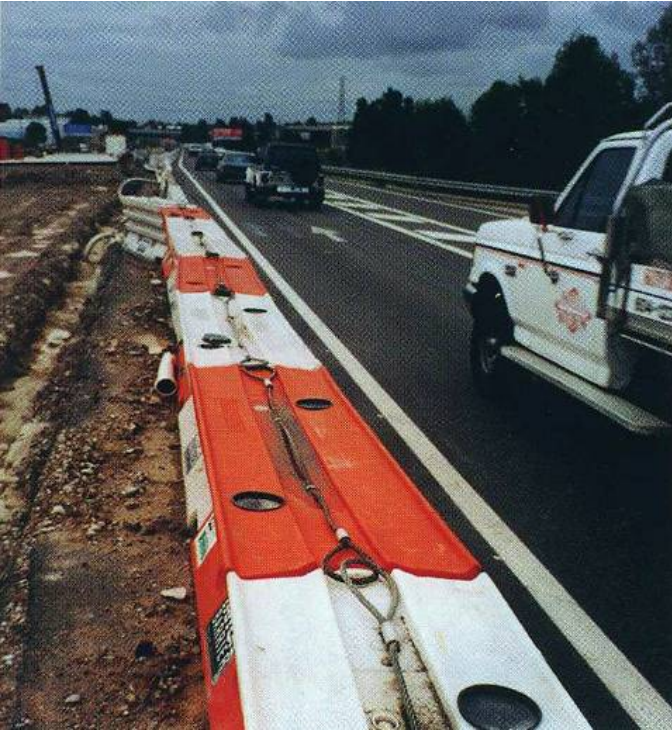
Figure 7.17: Blacked-out pavement lines and arrows are confusing especially at night-time; barriers overlapped incorrectly
