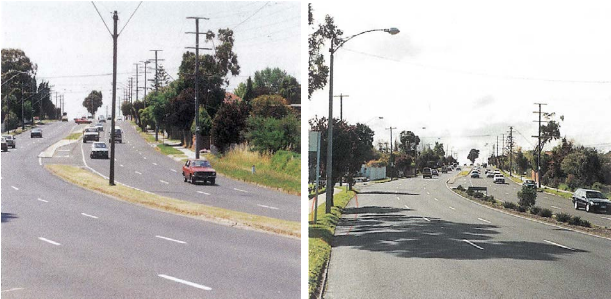
Figure 6.15: Non-frangible pole and the benefit of its removal
