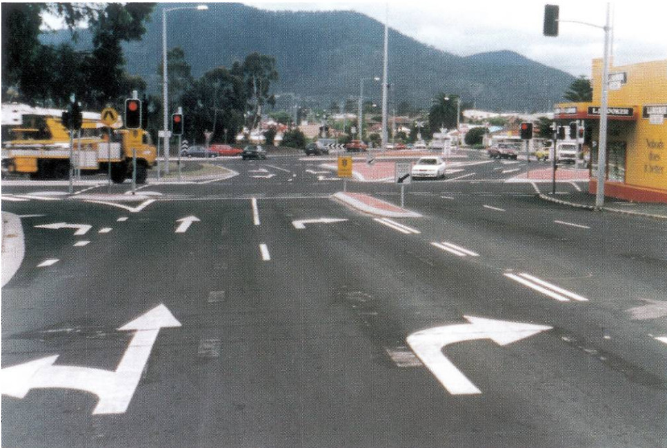
Figure 6.10: Confusing line markings
