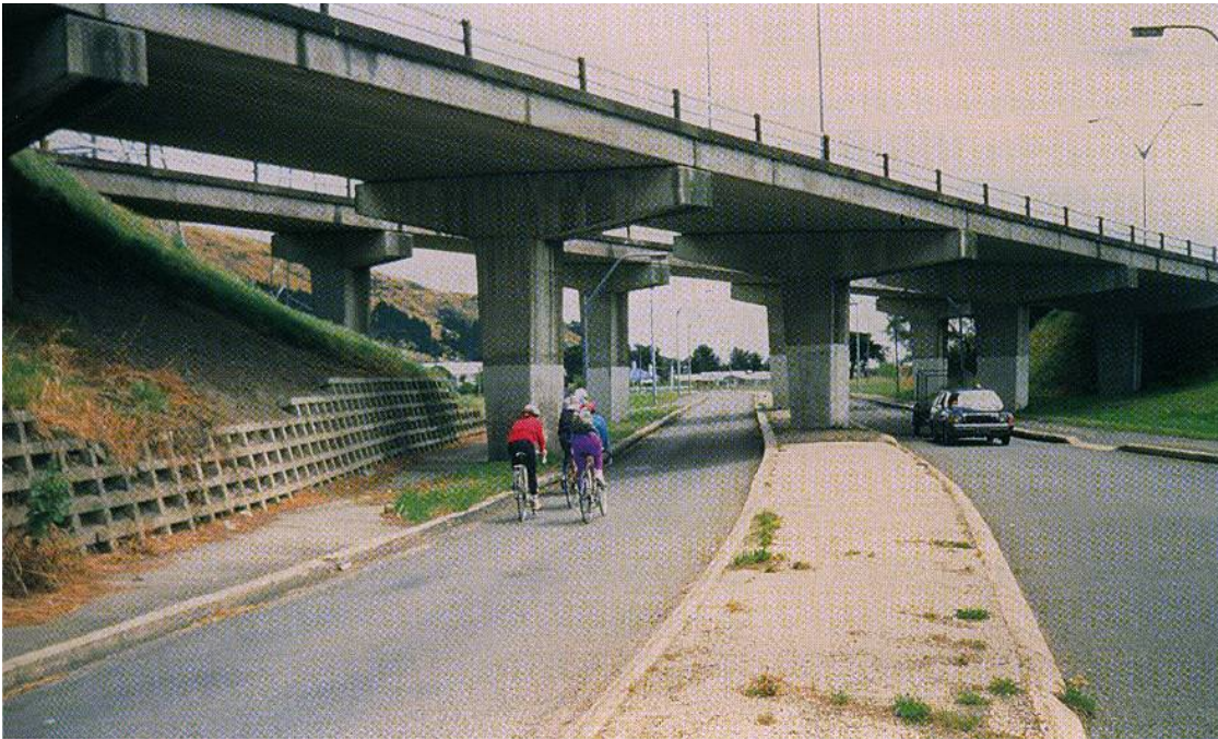
Figure 7.5: Bridge piers restrict forward sight distance at the location proposed for a new right turn
