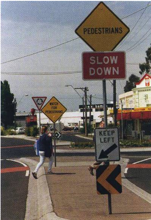
Figure 2.2: Adding signs is no substitute for safe initial design
