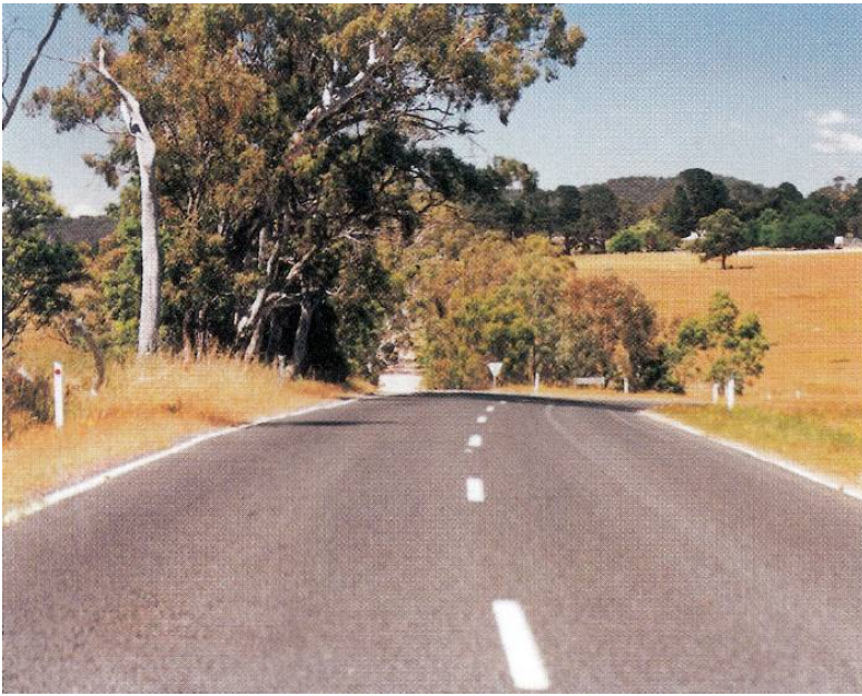
Figure 8.4: Visual cues such as lines of trees and driveway openings can suggest that a road continues straight when it actually takes a bend
