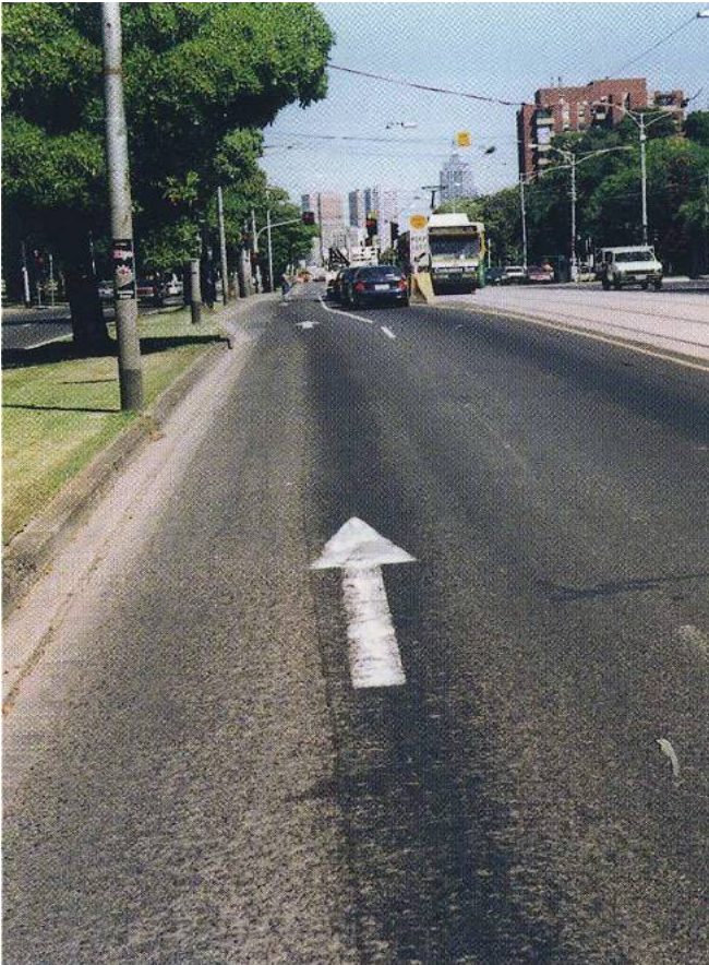
Figure 7.9: In Abbotsford Street the tram stop refuge will be extended over the striped area
