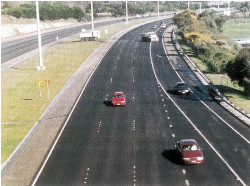
Figure 6.1: Potential hazard from movement of works traffic
