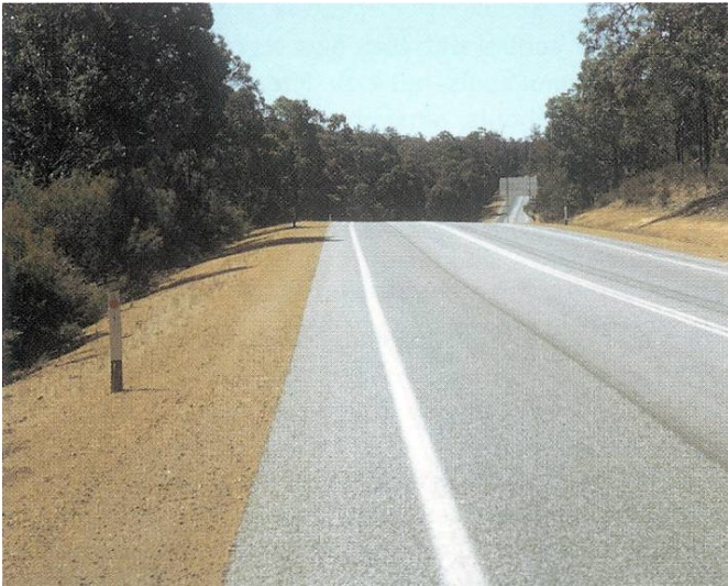
Figure 8.3: A summit vertical curve restricts the driver's view of the start of the horizontal curve and may produce a dangerous situation
