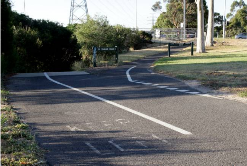
Figure 7.21: The link path from Toorak Road joins at an acute angle, with restricted sight distance
