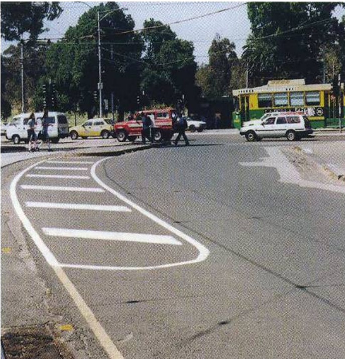
Figure 7.9: In Abbotsford Street the tram stop refuge will be extended over the striped area
