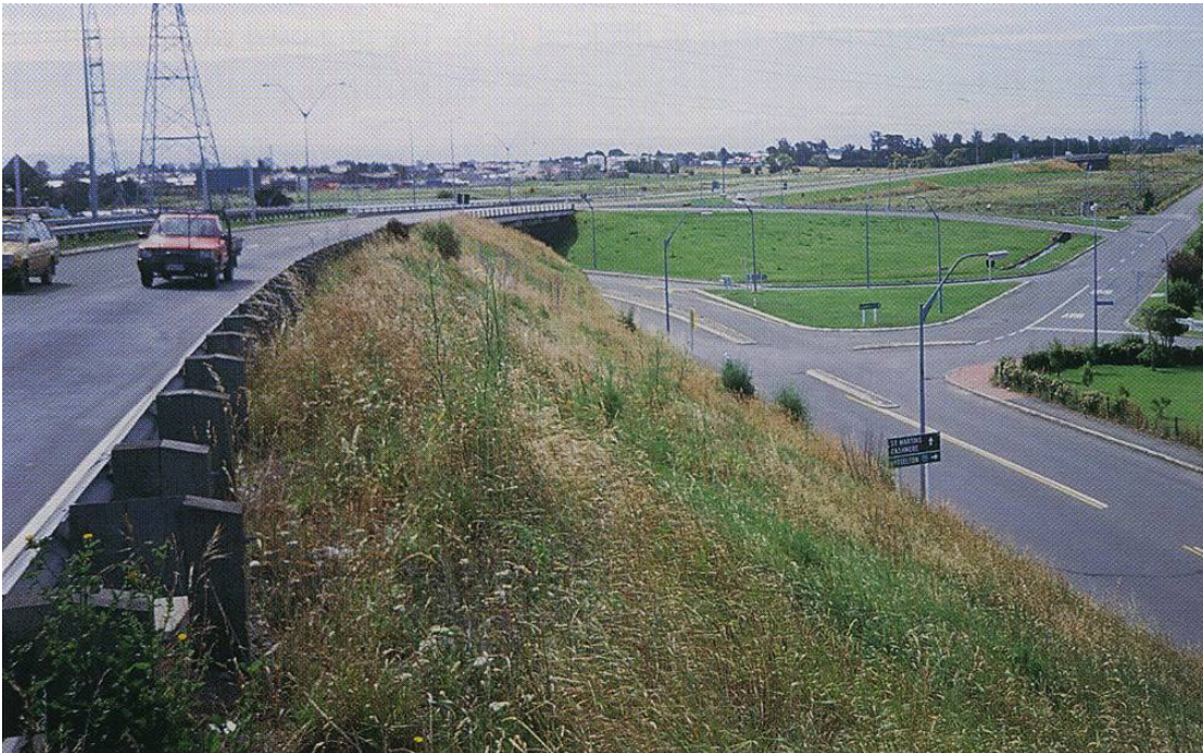
Figure 7.4: Limited area available for improving access onto Tunnel Road
