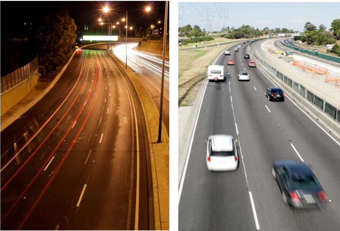
Figure 6.6: Three lane freeway without a full-width shoulder
