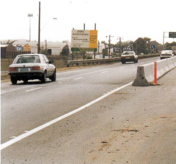
Figure 6.2: Unshielded barrier end
