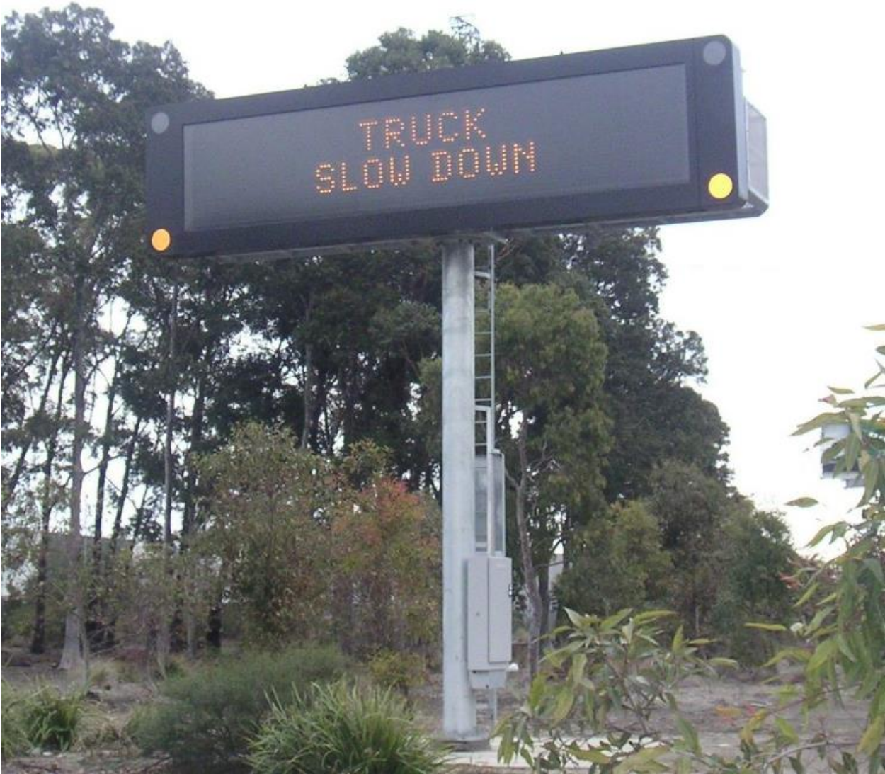
Figure 5.11: Vehicle activated warning sign for trucks
