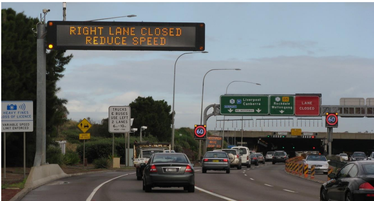
Figure 5.1: Cantilever-mounted VMS displaying a typical message
