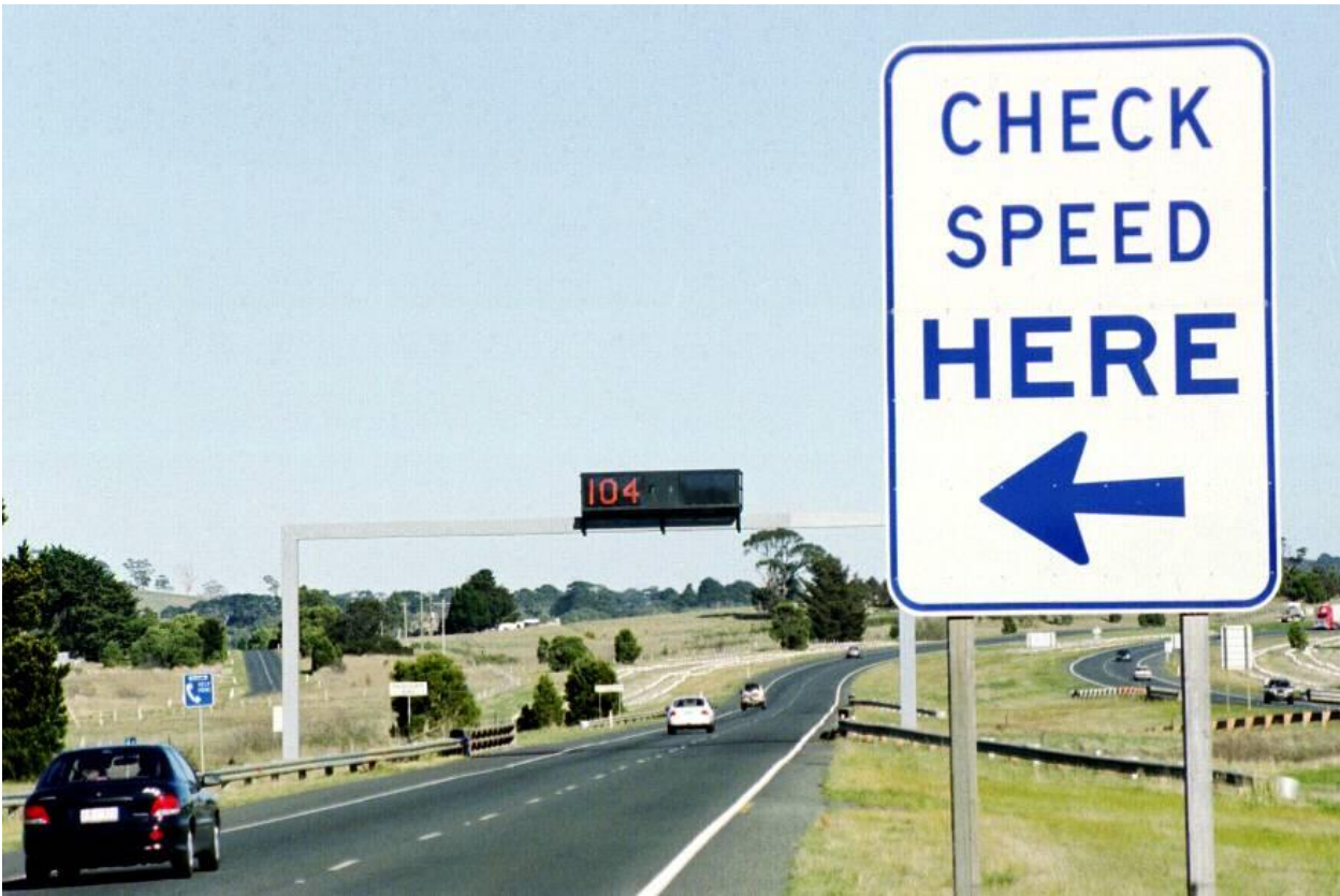
Figure 5.10: Speed indicator system on a motorway
