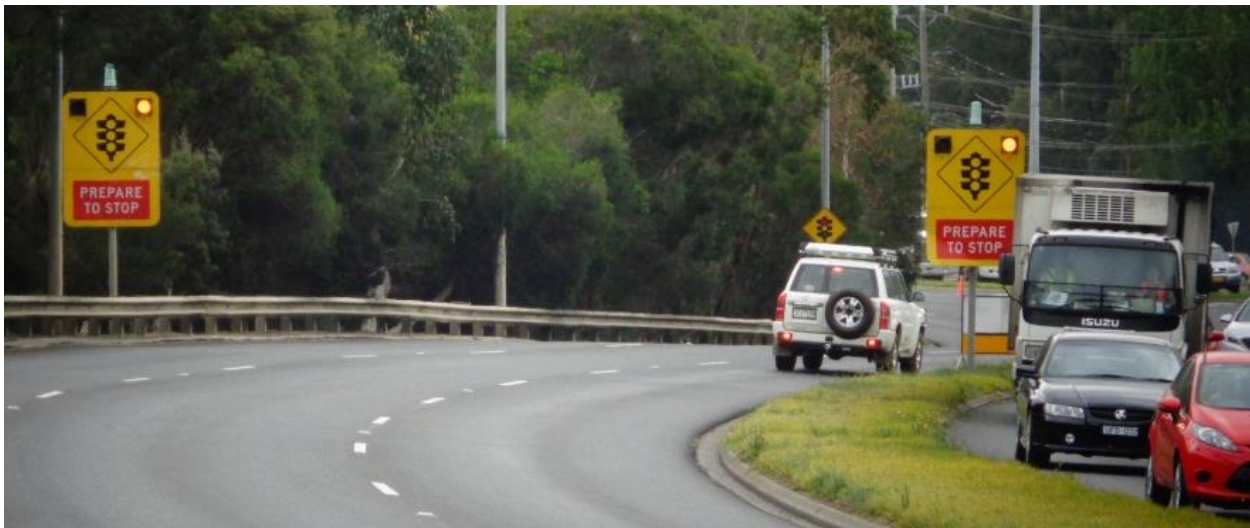
Figure 8.36: Advance warning signal signs in use
