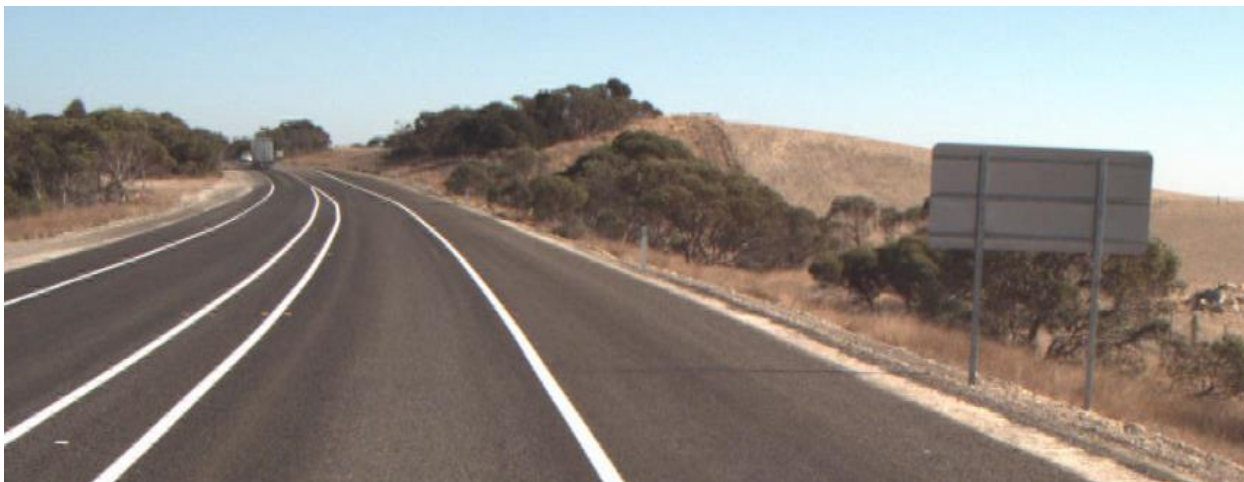
Figure 9.1: Wide centreline treatment example
