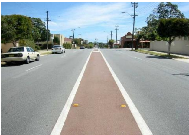
City of Subiaco, Western Australia
