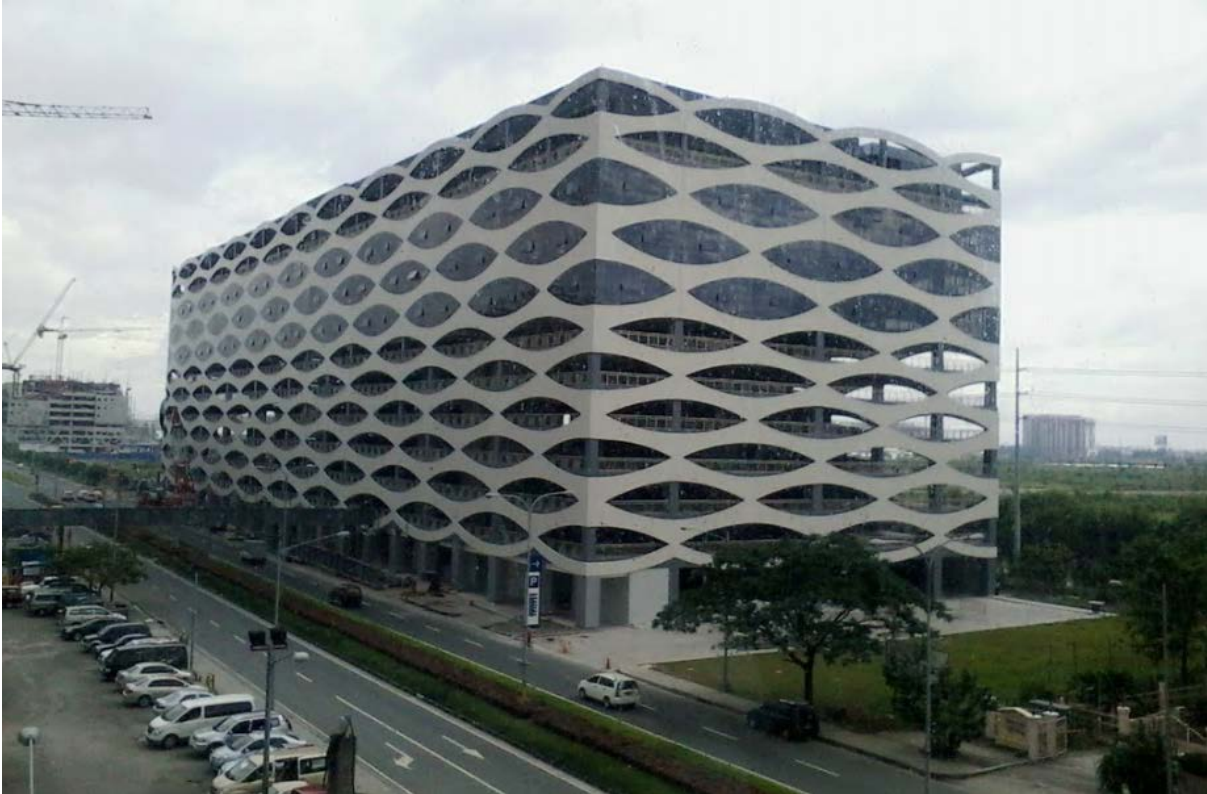
Figure 6.1: Example of aesthetically designed parking structure Manila, Philippines
