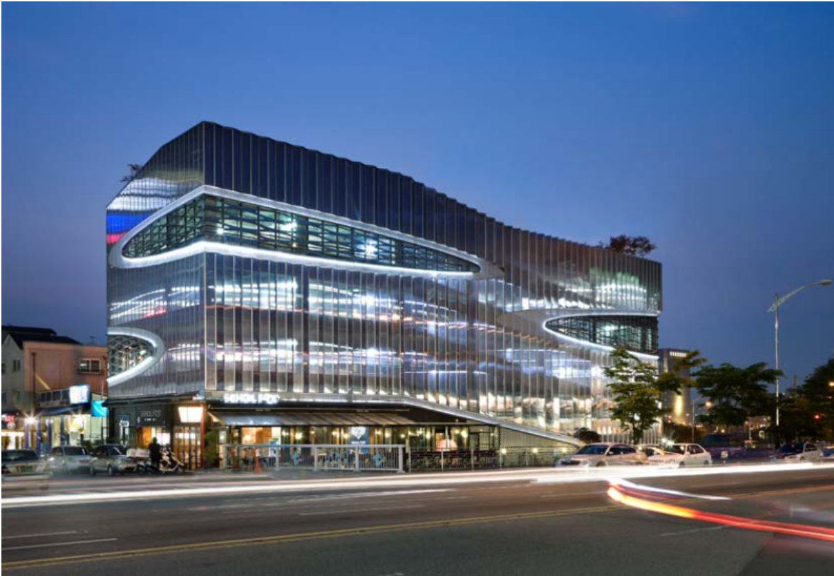
Figure 6.3: Example of aesthetically designed parking structure Seoul, South Korea
