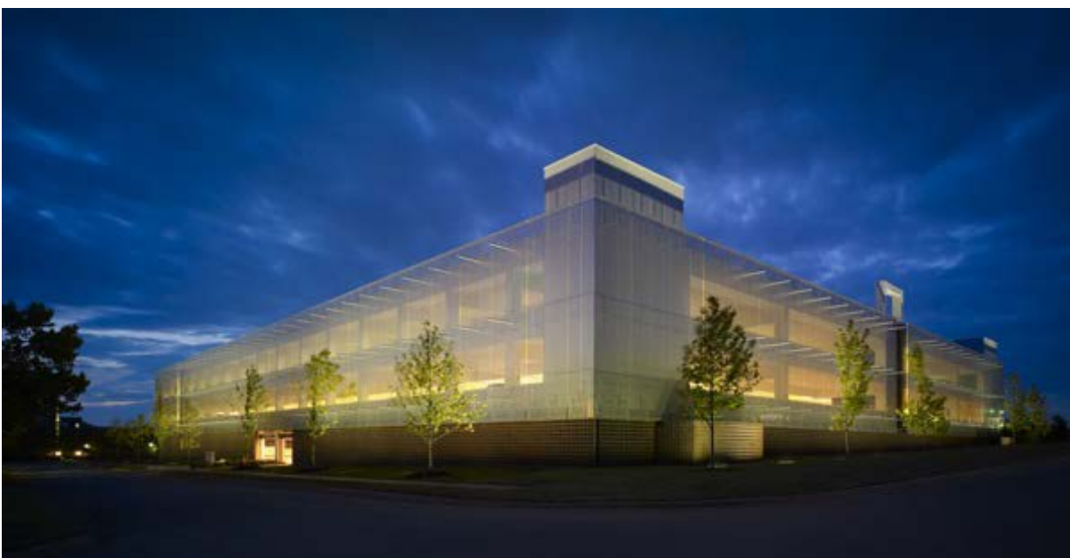
Figure 6.2: Example of aesthetically designed parking structure Oklahoma City, USA
