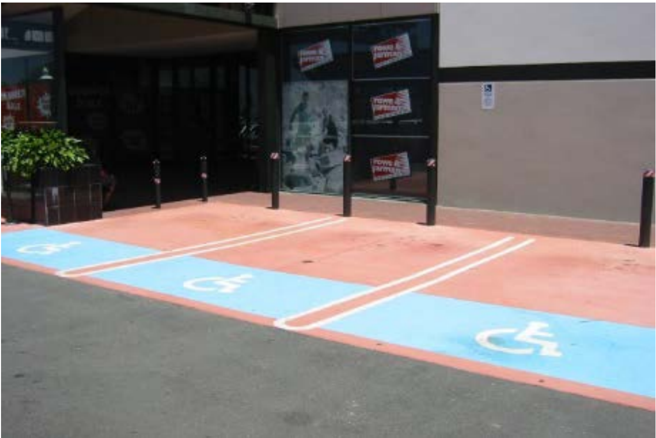
Figure 7.21: Example of a well-located parking bay for people with disabilities
