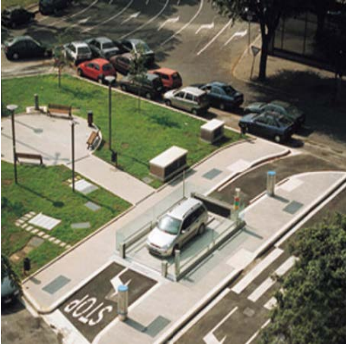
(a) Underground facility – Italy
