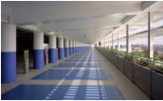
Figure 6.5: Example of well-designed pedestrian service elements inside parking structures California, USA
